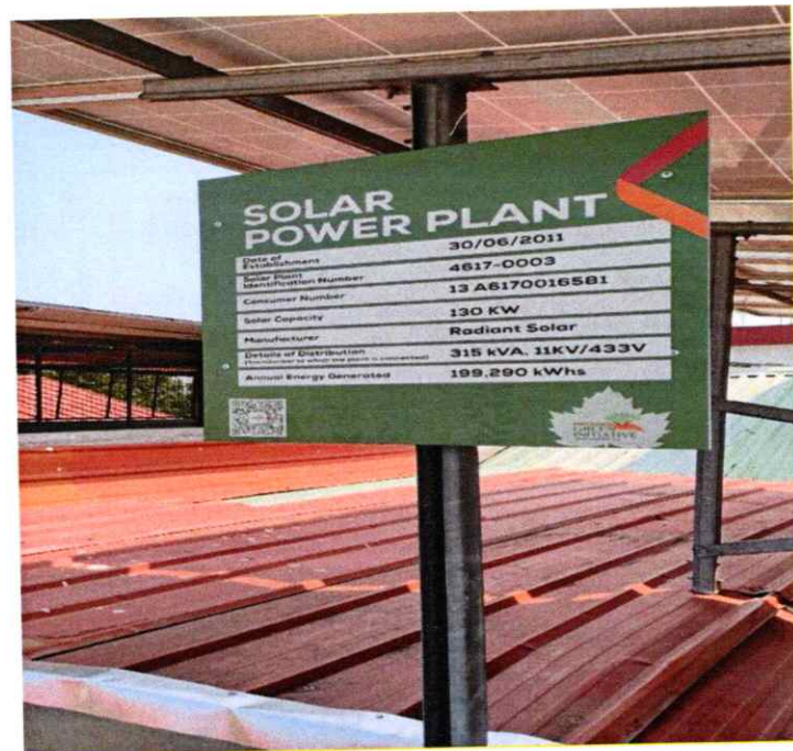
Solar Plant Specification
